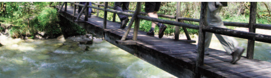
Footbridge © Matjaž Dovečar
